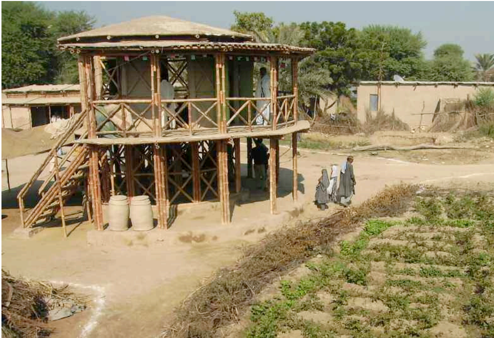
Left: Darya Khan Shaikh Village, Khairpur, Sindh. Flood resistant communal village hall on stilts, with permaculture of local vegetables surrounded by a dry brushwood fence that deters goats and cattle
