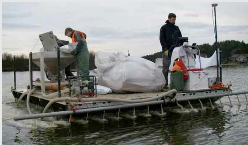
Applying the Phoslock treatment at Loch Flemington
